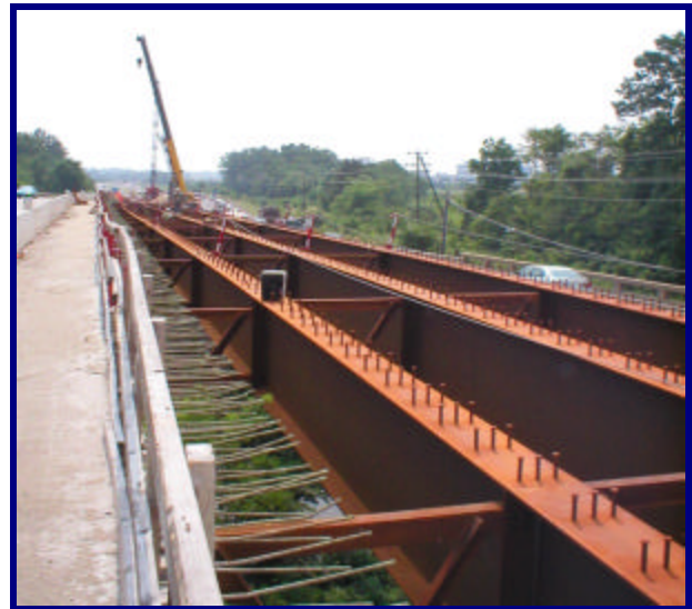
Westbound Route 625 Bridge over Broad Run after steel erection.
