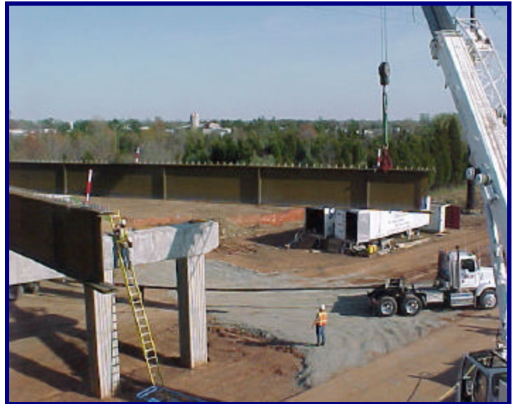
Structural steel erection for the Air & Space Parkway Bridge over Route 28
