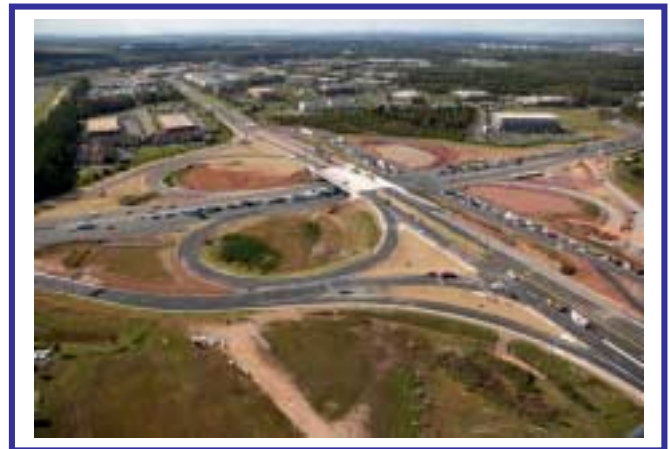
The Route 606 Interchange opened to public on October 9, 2004
