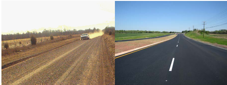
Loudoun County Parkway was a two-lane gravel road before its widening to four lanes
